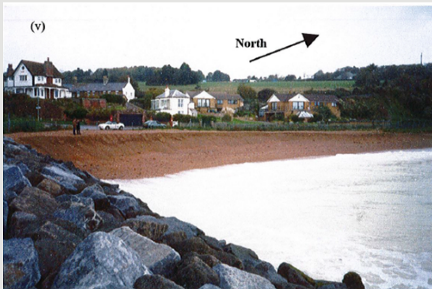
(v) This is Oldstairs Bay in September 2000. In the background is the housing and the road endangered by the advancing sea. In the foreground is the rock revetment built to replace the metal wall. During the 30 months since the storm the bay has retreated about 40m, despite the revetment.
