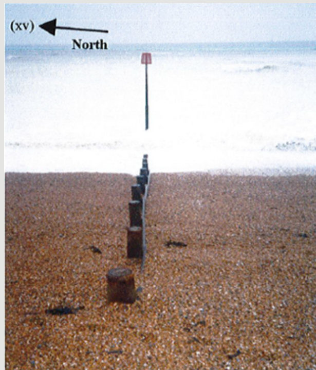
(xv) This is the same groyne (at high tide) in August 2000. Southward movement of material due to longshore drift has overwhelmed and buried relatively new groynes.
