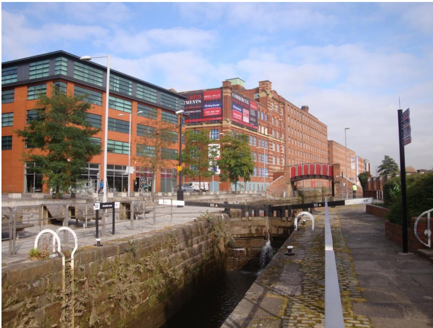
A modern photograph of the former cotton mills and Rochdale Canal, Redhill Street.
